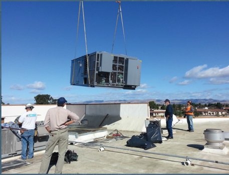
▲ The old MZ unit being uninstalled and preparing the site for the new unit.
