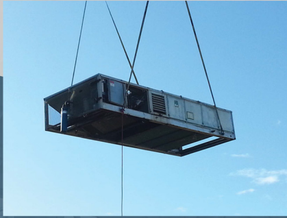
▲ The old MZ unit being uninstalled and preparing the site for the new unit.
